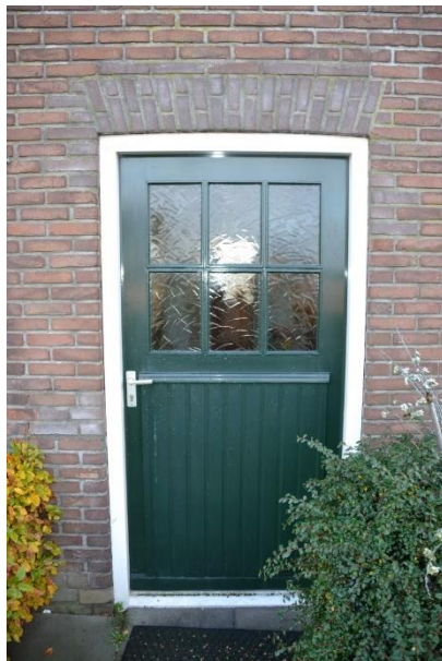
Later aangebrachte deur in de vm. stal.
