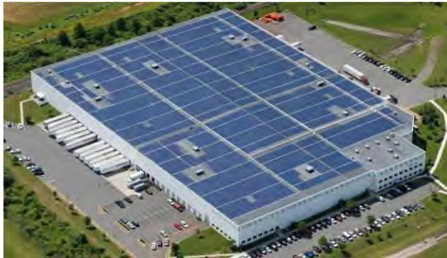
Local energy production
