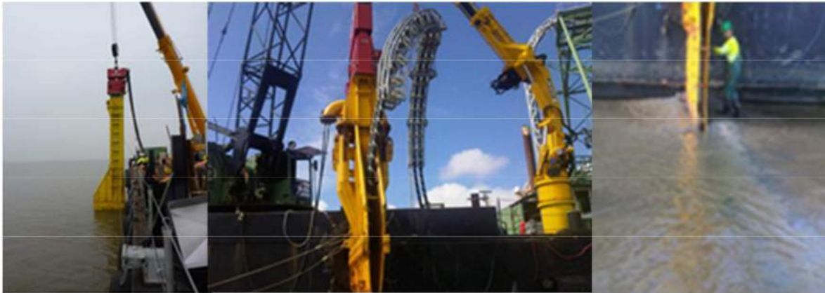
Figure 50 Vibration plough deployed from a barge
