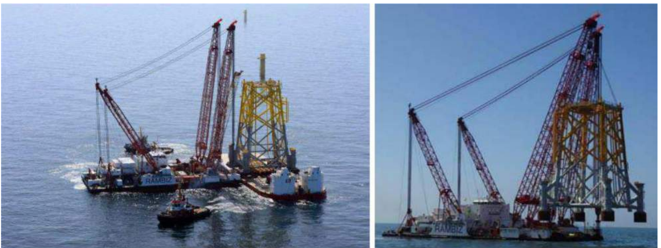
Figure 58 Installation of jacket
