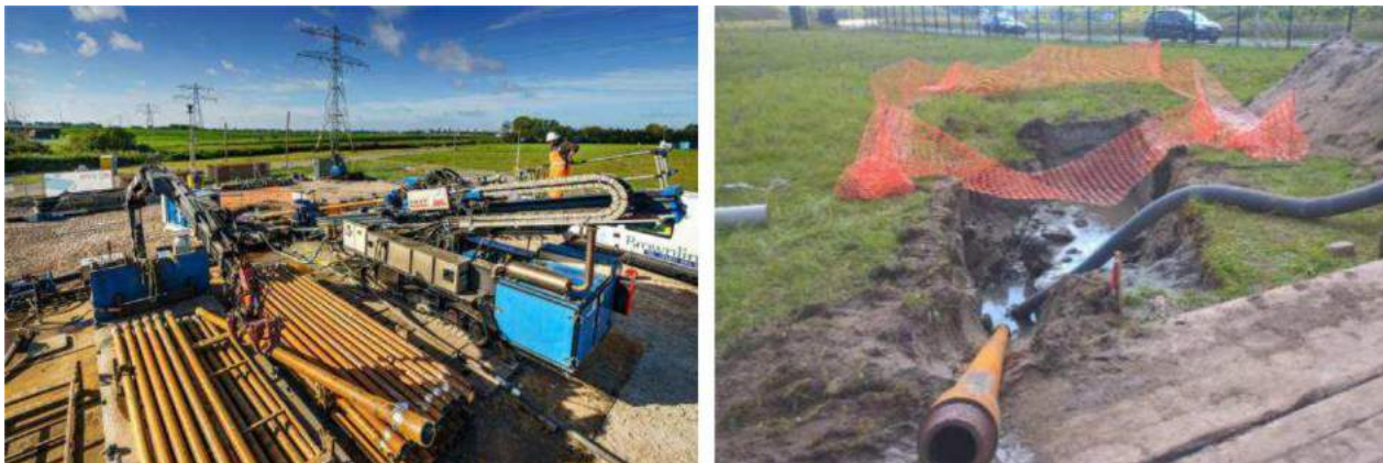
Figure 26 Example of HDD entry and exit point
