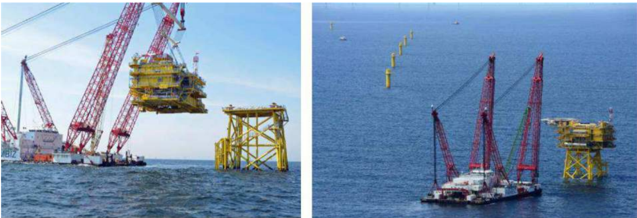
Figure 60 Installation of topside
