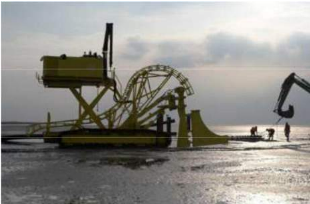
Figure 51 Vibration plough on tracks
