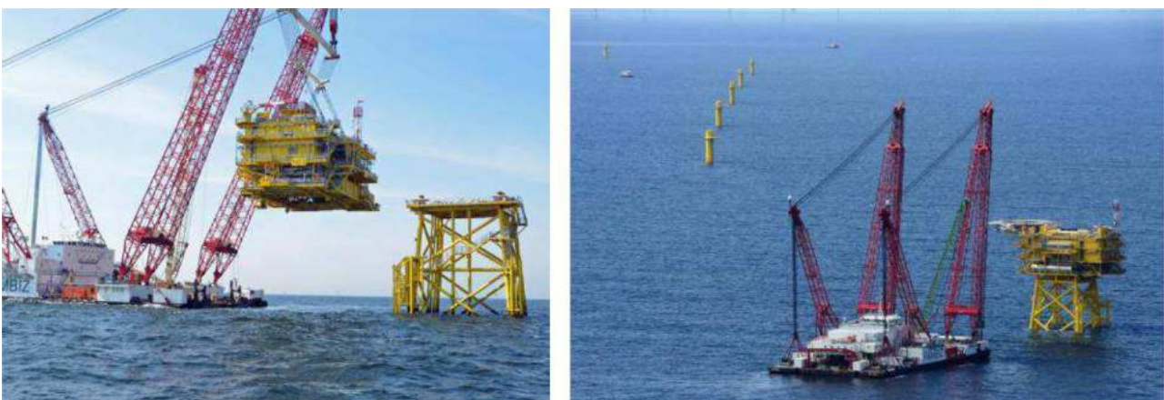
Figure 60 Installation of topside
