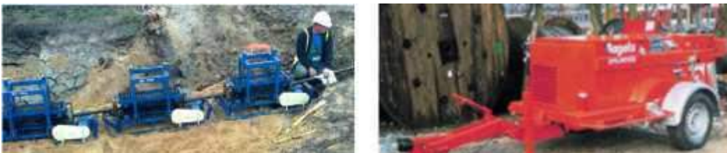
Figure 17 Typical cable tensioners (left) & cable winch (right)
