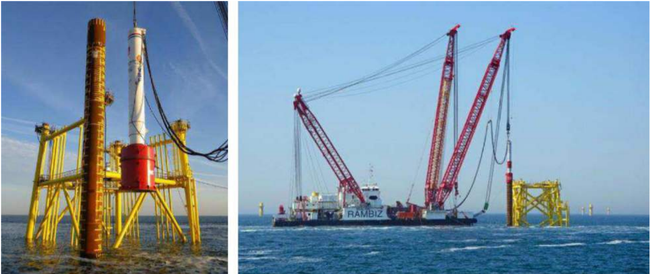
Figure 59 Piling of jacket
