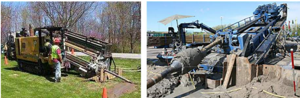
Figure 29 Example HDD rigs - [left] midi rig - [right] maxi rig
