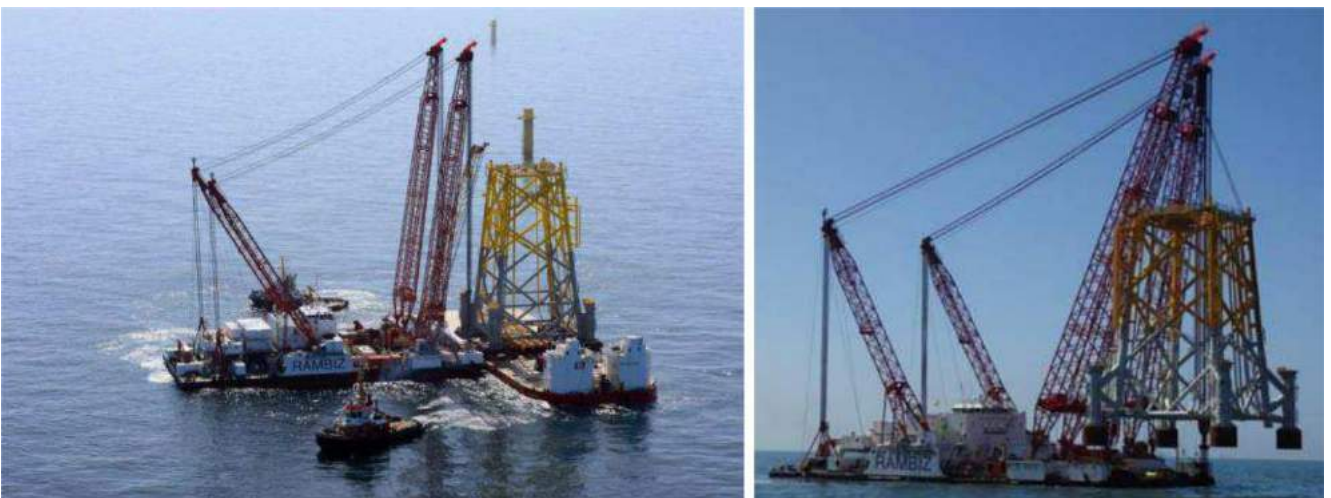
Figure 58 Installation of jacket
