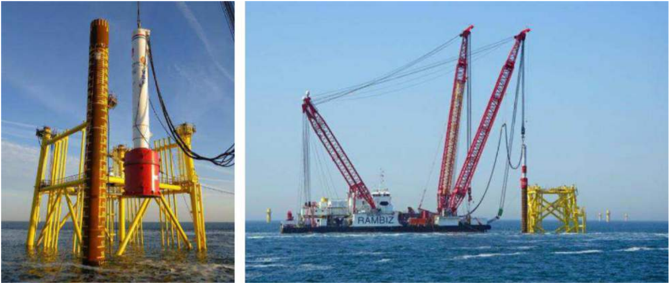
Figure 59 Piling of jacket
