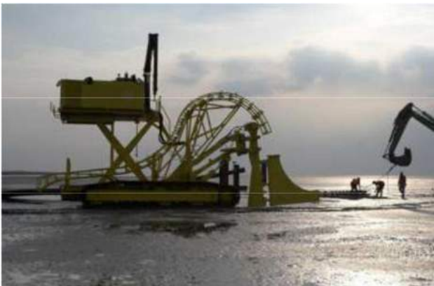
Figure 51 Vibration plough on tracks
