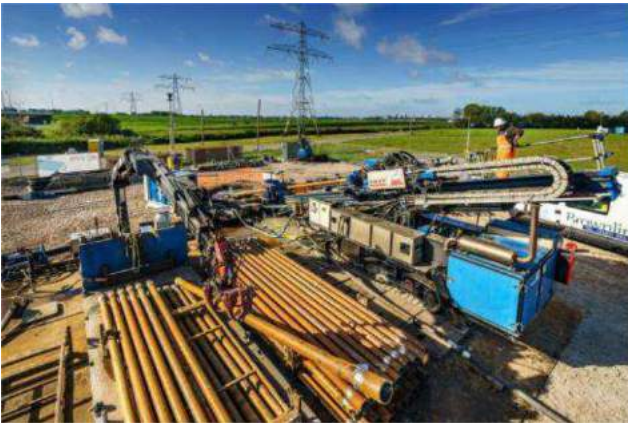
Figure 26 Example of HDD entry and exit point
