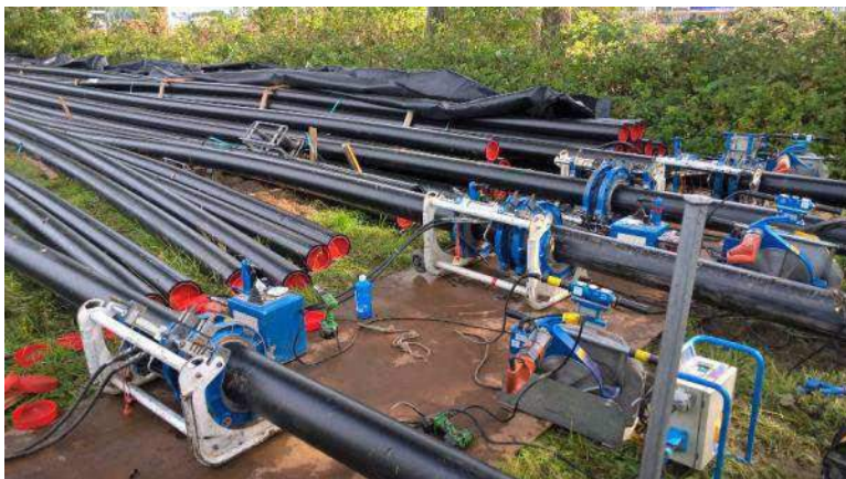
Figure 27 Welding of HDPE ducts
