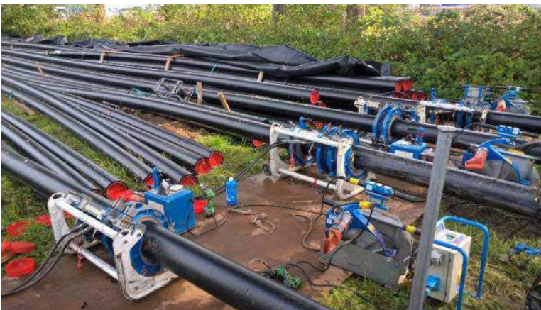
Figure 27 Welding of HDPE ducts
