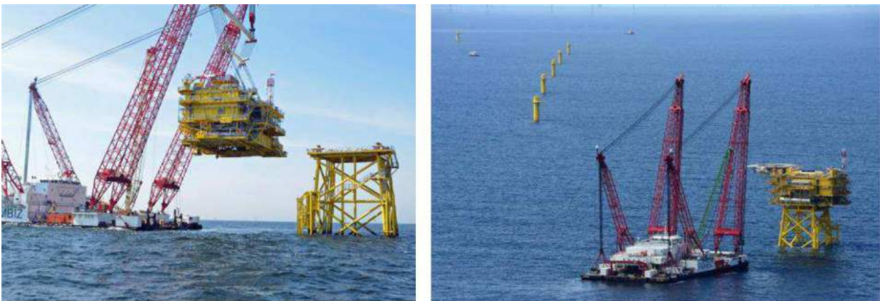
Figure 60 Installation of topside
