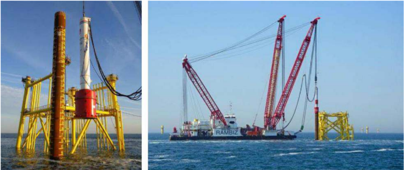
Figure 59 Piling of jacket
