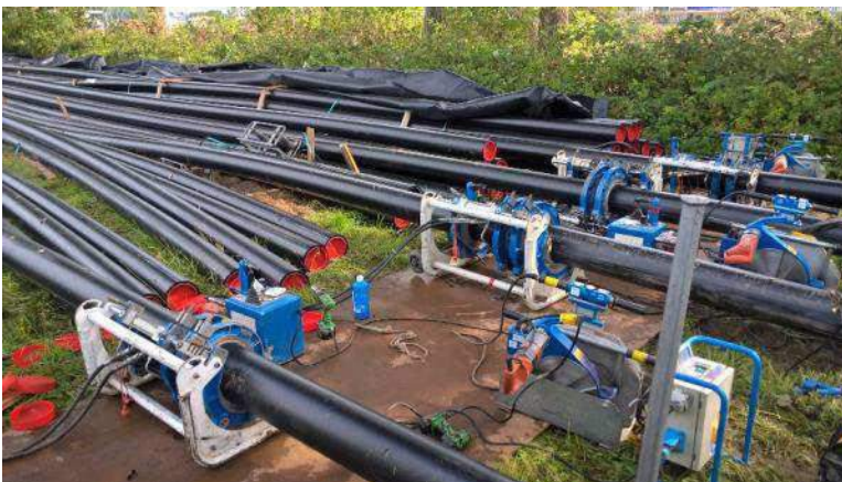
Figure 27 Welding of HDPE ducts
