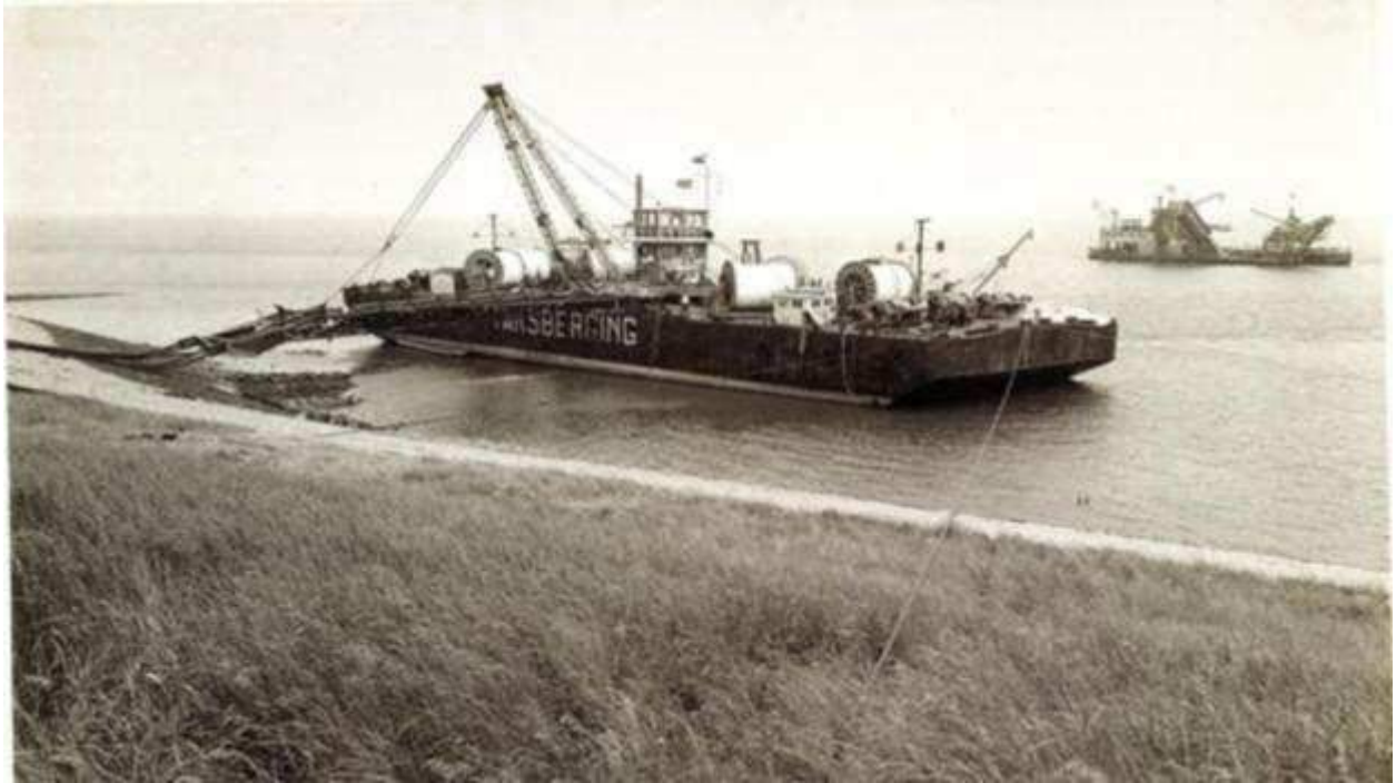
Figure 48 Cable installation by a vertical injector like trencher in Zeeland
