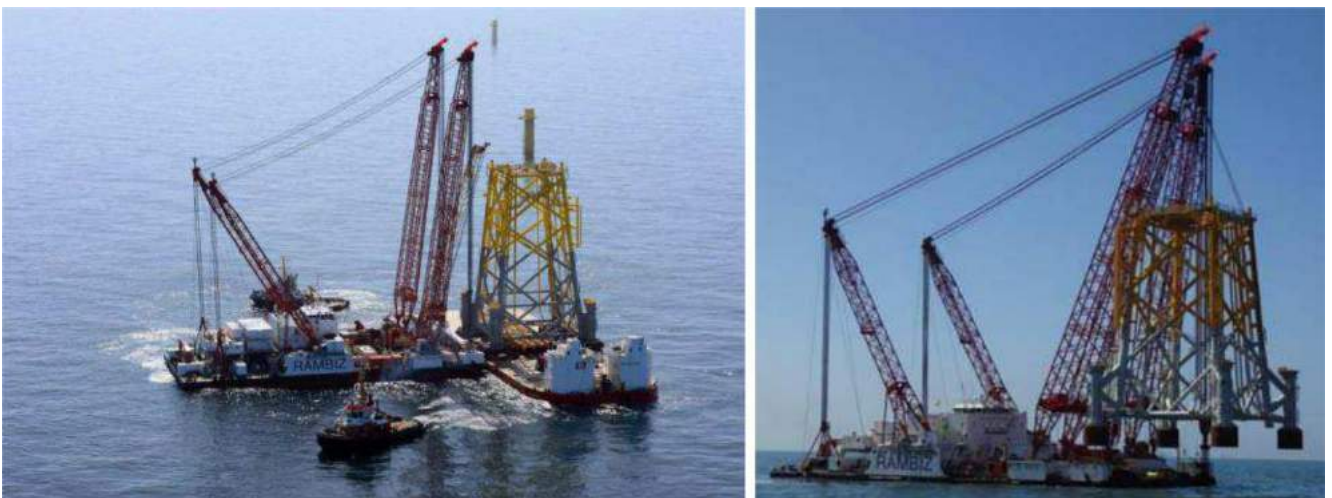
Figure 58 Installation of jacket
