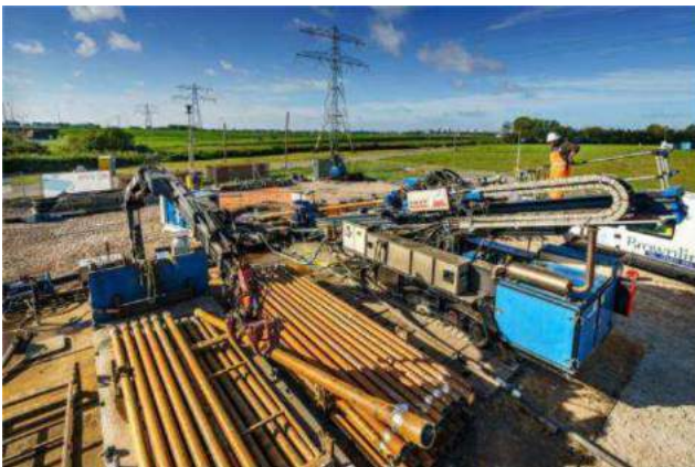
Figure 26 Example of HDD entry and exit point
