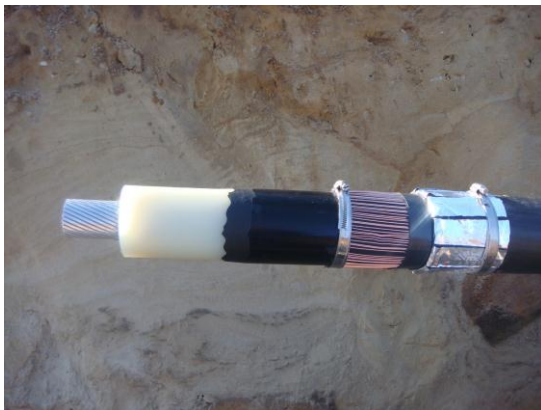
Figure 3: Typical HVAC cable
