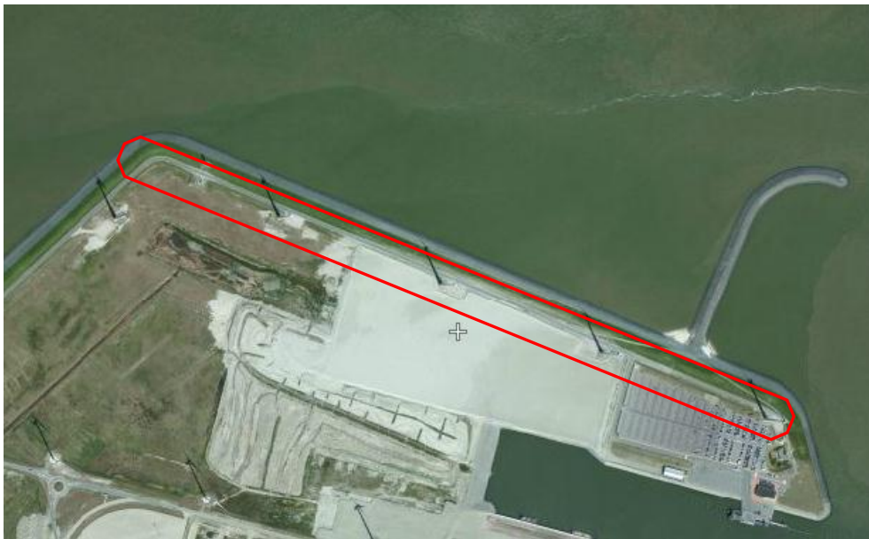
Figure 13: Overview Western side Eemshaven
