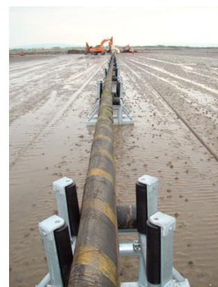
Figure 14: Cable on rollers
