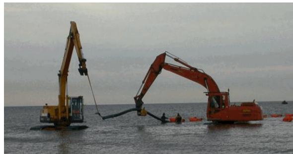
Figure 16: Excavator with lifting bow, removal of floaters
