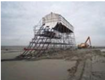
Figure 29: Typical example Shallow water Jointing platform
