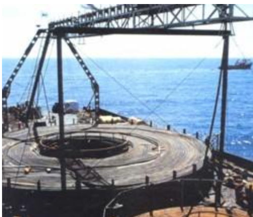
Figure 10: Cable on board a shallow draught installation barge
