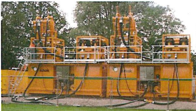
Figure 38: Bentonite Mix installation
