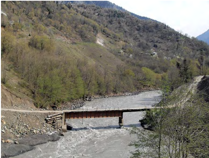
Photo 16. Sediment supply towards the Enguri river due to road construction.
