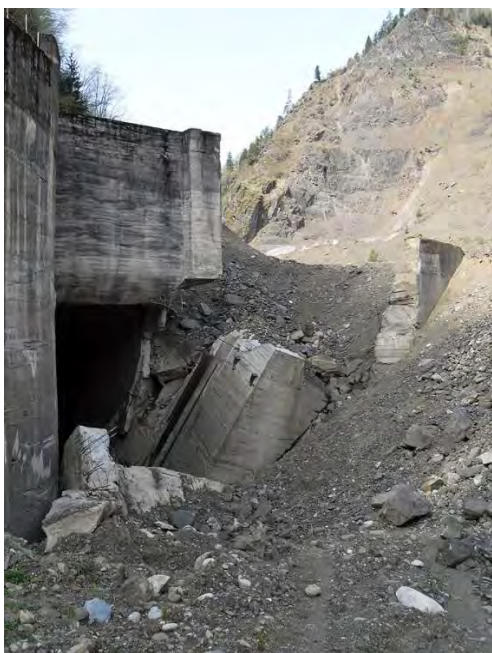
Photo 13. Collapsed inlet of river diversion tunnel
