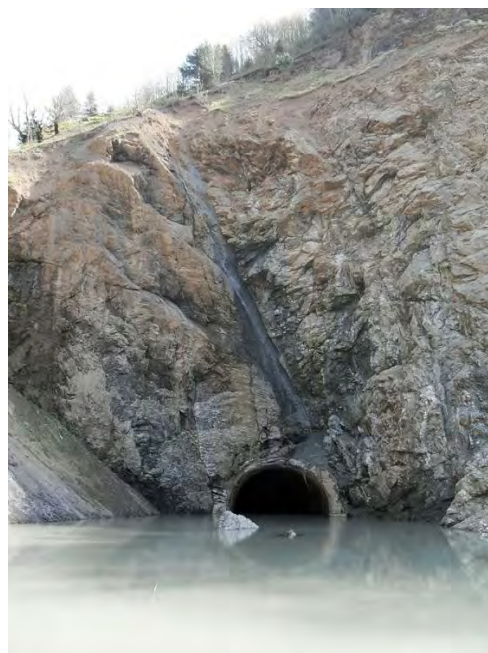
Photo 14 Landslide due to erosion at outlet of river diversion tunnel.
