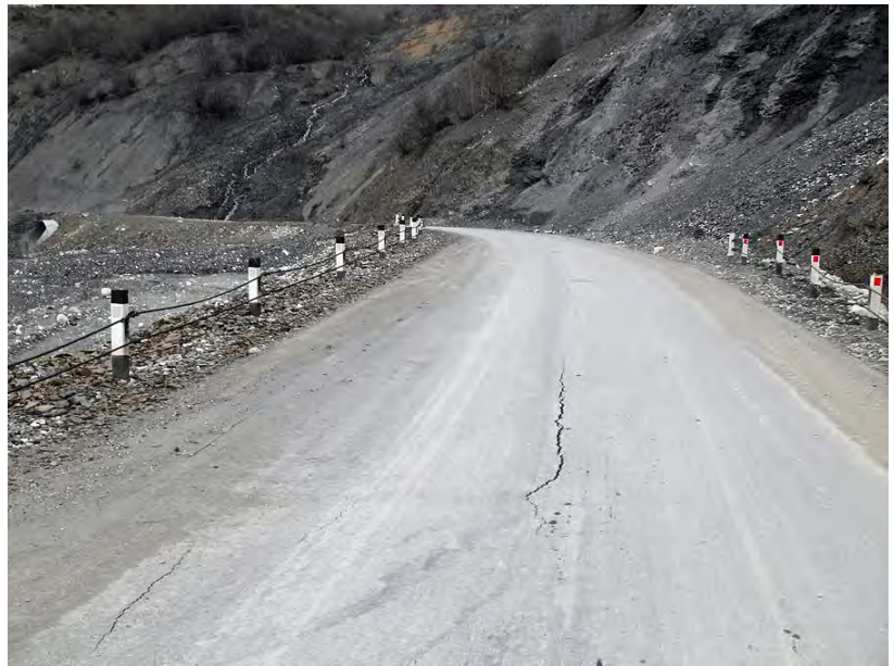
Photo 19. In sufficient road drainage cause instability in the road foundation and leads to landslides.
