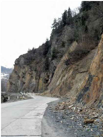
Photo 18. Also rocky slopes can be instable and yield sediments.
