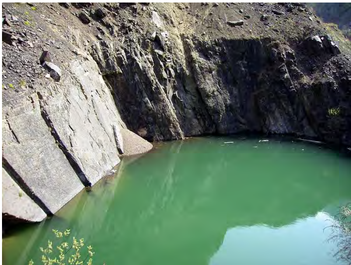
Photo 13. Collapsed inlet of river diversion tunnel
